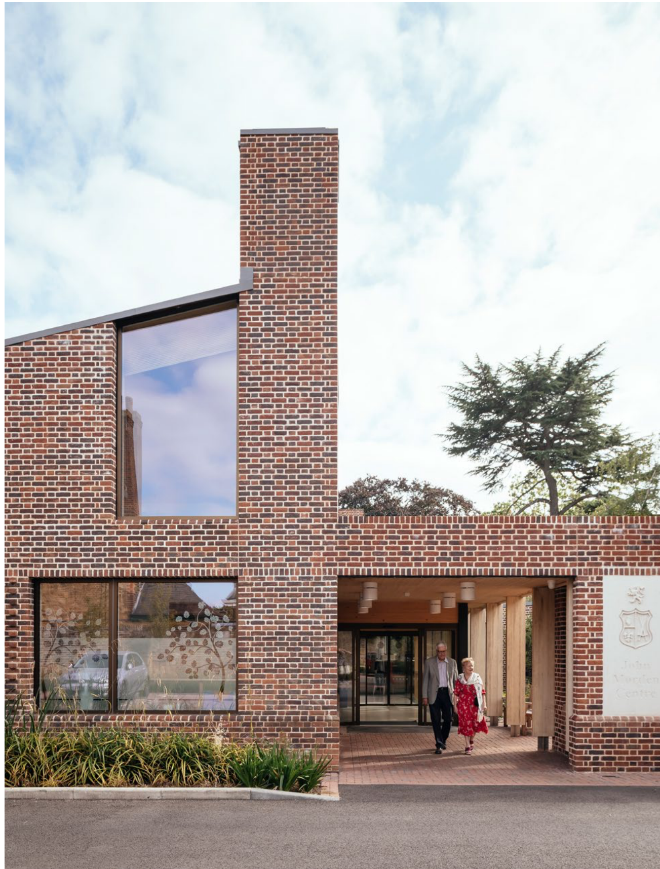
Brick external facing suits the listed building setting
